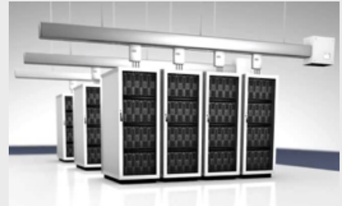
FIGURE 4: OVERHEAD BUSWAY IN DATA CENTER EXAMPLE
